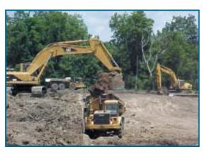
**Item 477L** - The Notice to Proceed was granted to ASA Enterprises of Jackson, MO on August 1, 2002. This is a 5.1 mile conventional levee enlargement project. Relief Wells were installed in 1997, therefore a berm is not needed.
